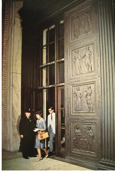
Figura 1 - Massive sliding bronze doors of the supreme court building in Washington, D.C.
